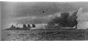
The Bismarck has turned to starboard of her cruiser consort. Her guns trained astern, she has just fired a salvo. To the right, is the smoke from a previous salvo and a column of water from one of the Prince of Wales 's 14-inch shells. The splash of a major-caliber projectile could easily reach seventy meters in height. (Photograph courtesy of Paul Schmalenbach.)
